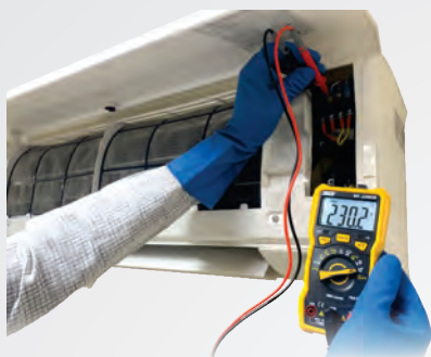
Check AC Voltage of Indoor Unit
